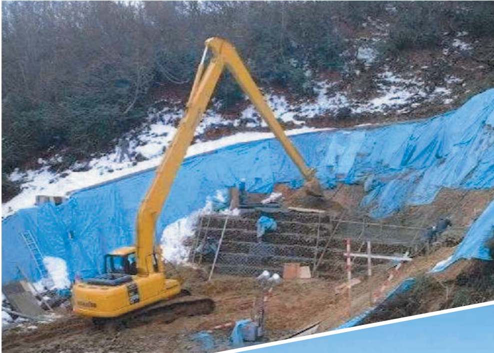
■ For work of light duty (PC200LC handling construction materials)
